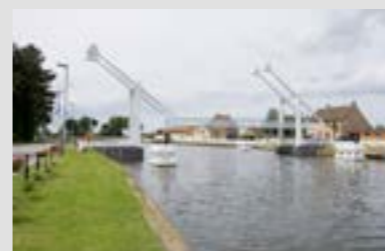
mobile brug, Stalhille
